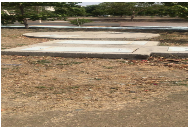
Ground water recharge wells
